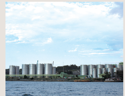
View of Kutai Refinery Nusantara in East Kalimantan, Indonesia from the sea
