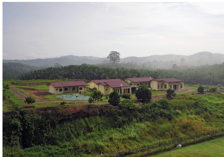
Employee housing complex at PT Fortius in Jambi, Indonesia
